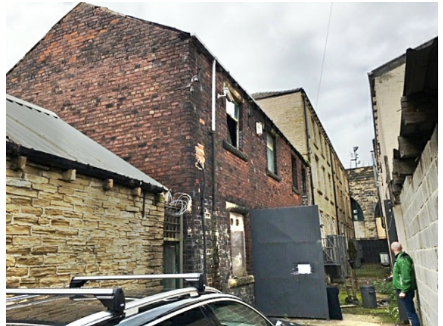
View from service access
