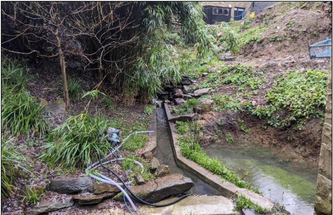
Plate 2. Concrete channel carrying stream near northwest corner of swimming pool, noting small pond (to right of image) formed by leaking concrete channel
