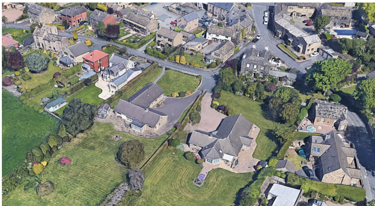
Image 3 - Existing Aerial View 1
