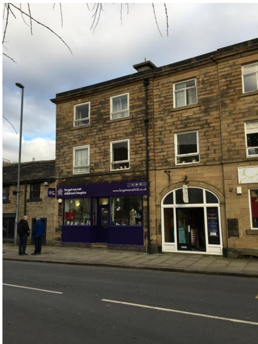
Figure 1: West Elevation (pre 2018 replacement windows)
