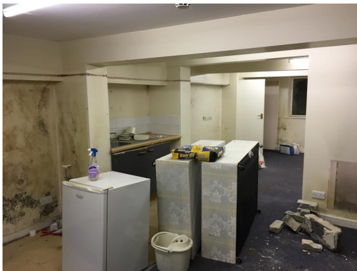
Figure 7: Basement unused office
