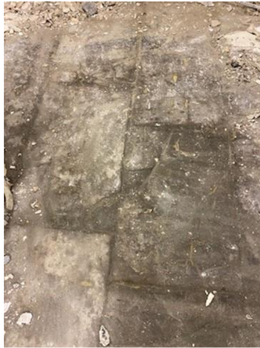
Figure 9: Stone flag floor in basement
