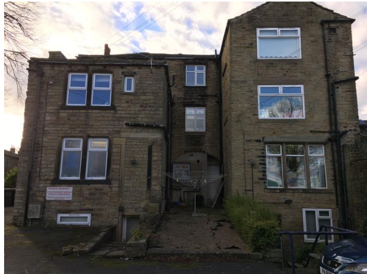
Figure 4: Eastern Elevation (pre 2018 replacement windows)
