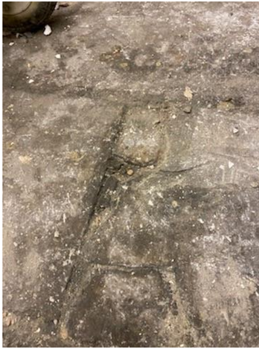
Figure 8: Stone flag floor in basement
