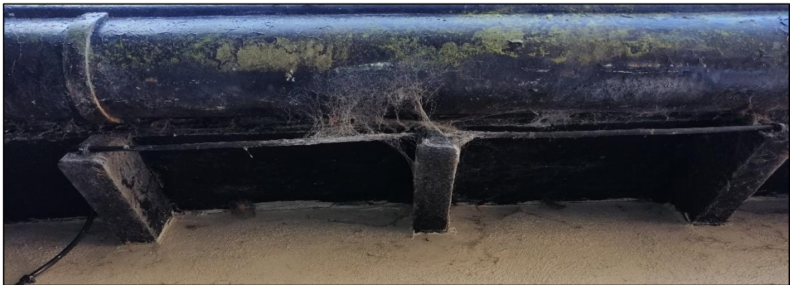
Plate 4. Directly inspected feature, as indicated by red symbols.
