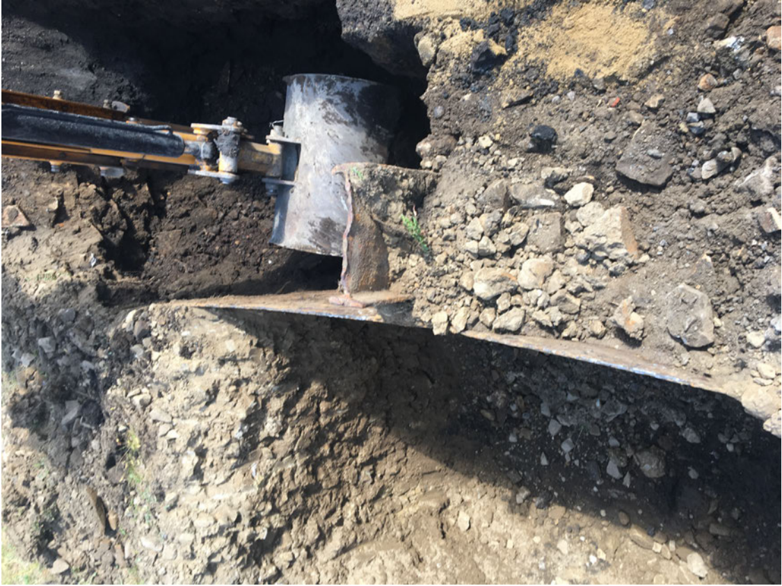
Photo 1 – Gas Holder 2 metal frame and stanchion
