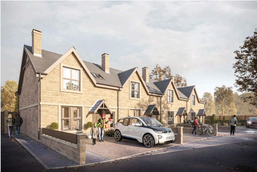
View of new terrace facing Bierley Marsh
