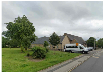
Primary School extensions
