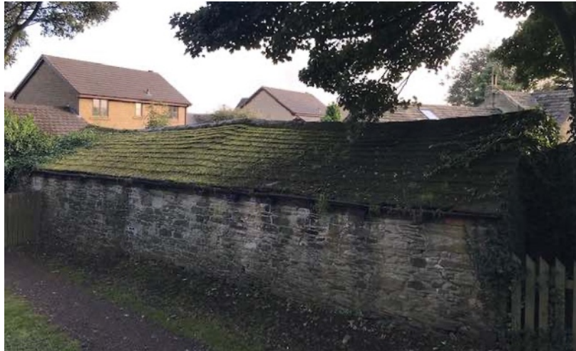
Example of a wall forming enclosure and screening on Bierley Marsh
