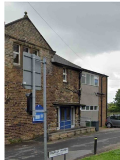
Brickwork of St Luke's
