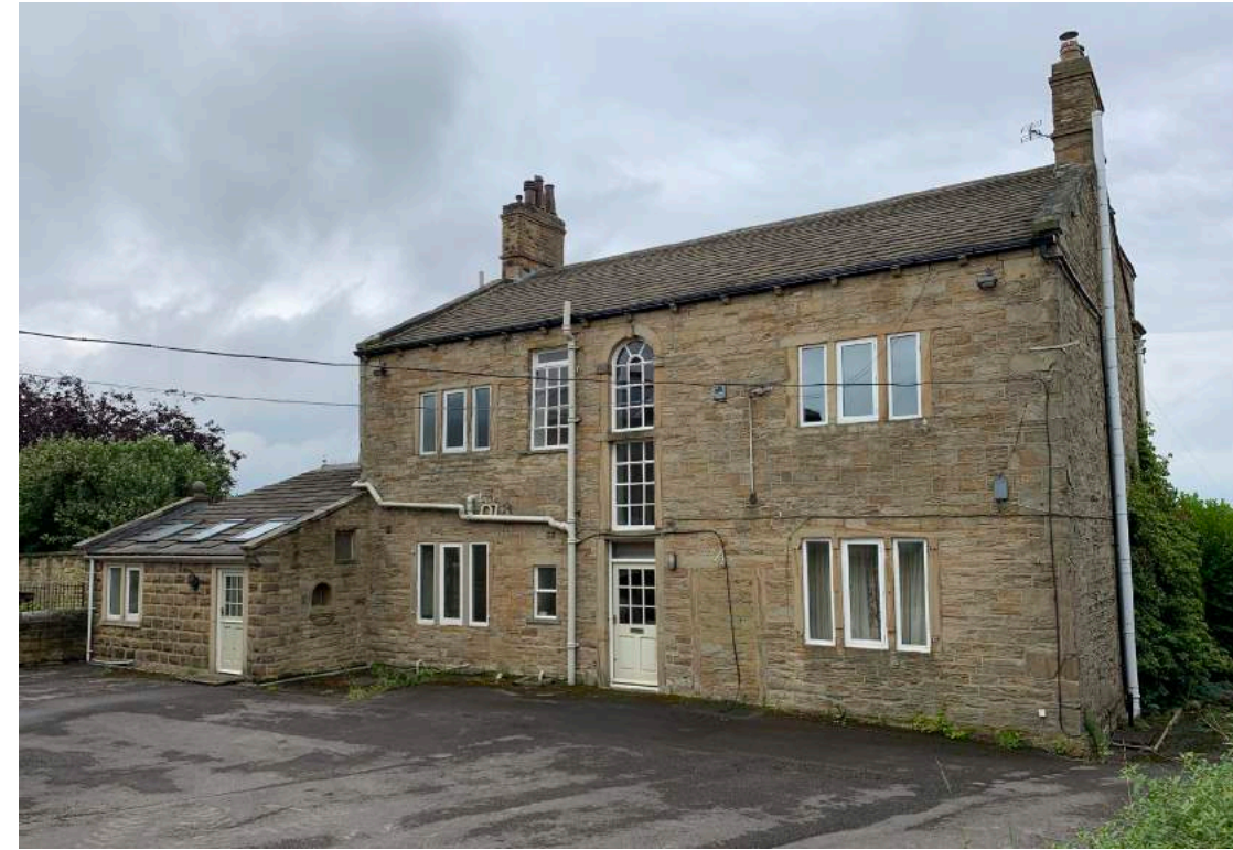
Figure 5 – View of the rear of Clough House
