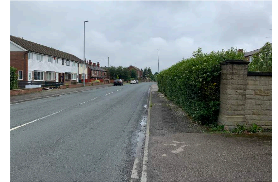
Figure 2 – Existing footway on Leeds Road towards Birstall
