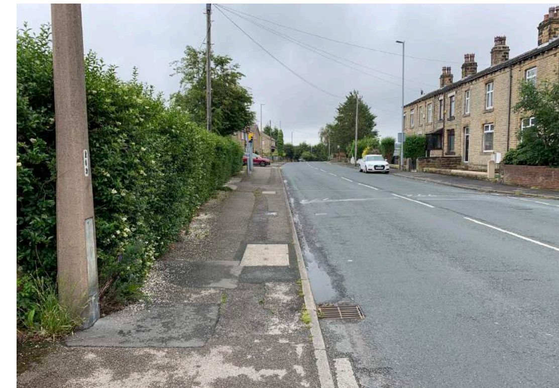
Figure 3 – Existing footway on Leeds Road towards Morley
