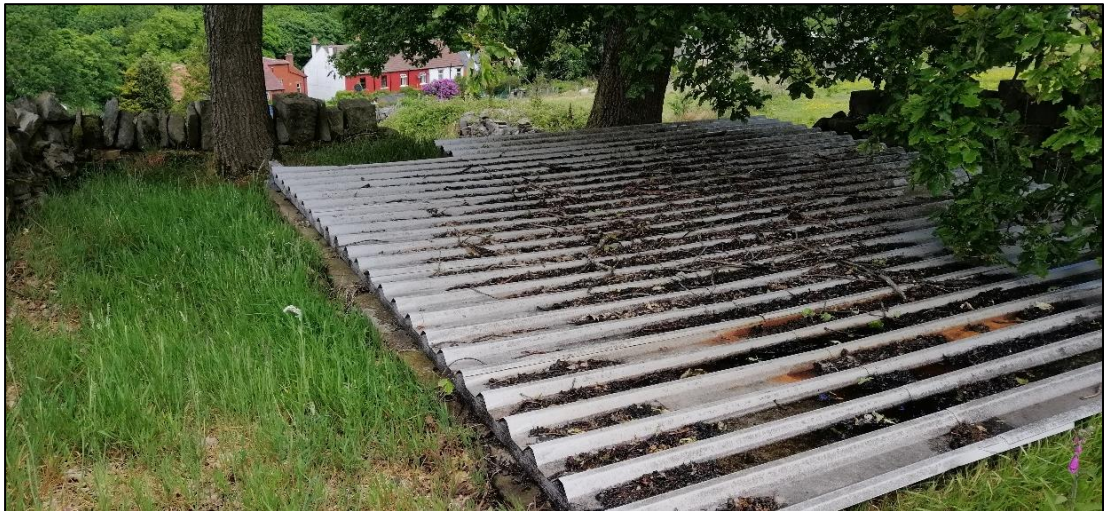
Plate 11. Water storage tank
