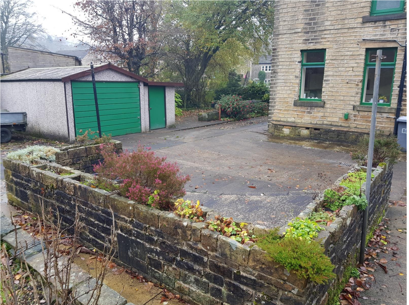
Existing hardstanding where the extension is proposed
