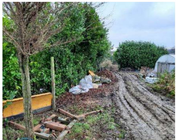
Photograph 22: View looking north west along the bare ground and H1
