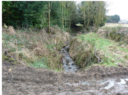
Existing culvert with ditch flowing south off-site
