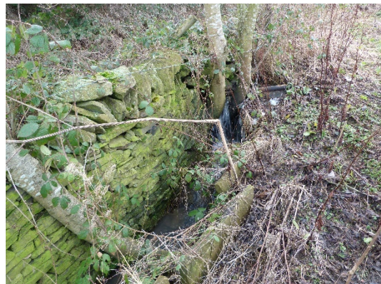
Location where channel runs under wall (switches from west of wall to east of wall).
