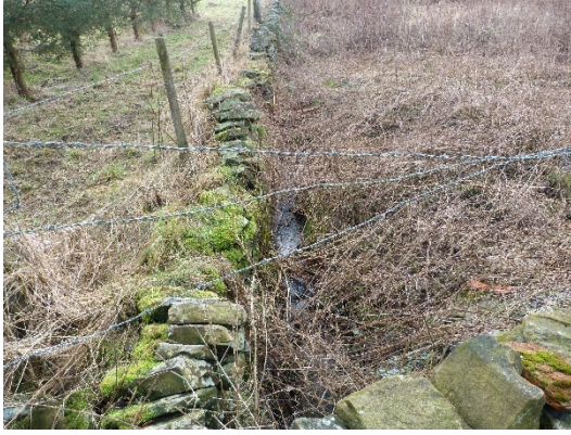
Northern end (junction with roadside wall)
