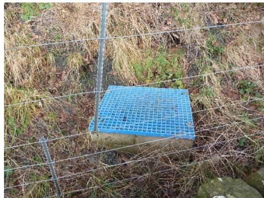
Drain to north of site (across road) into which ditch terminates.
