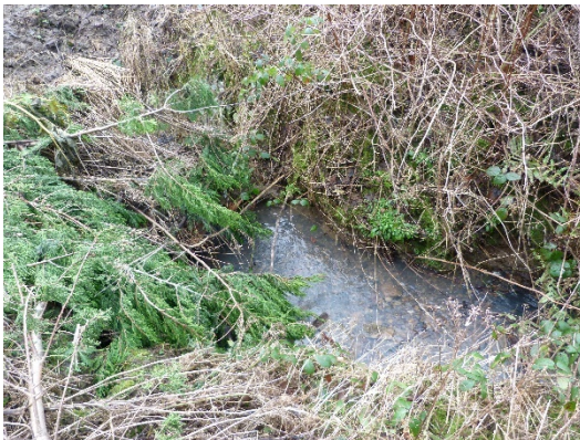
Ditch just north of existing culvert
