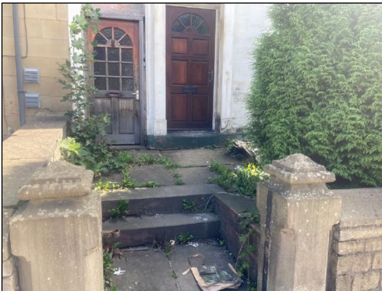
View showing the steps up to front door plate relative to the pavement level
