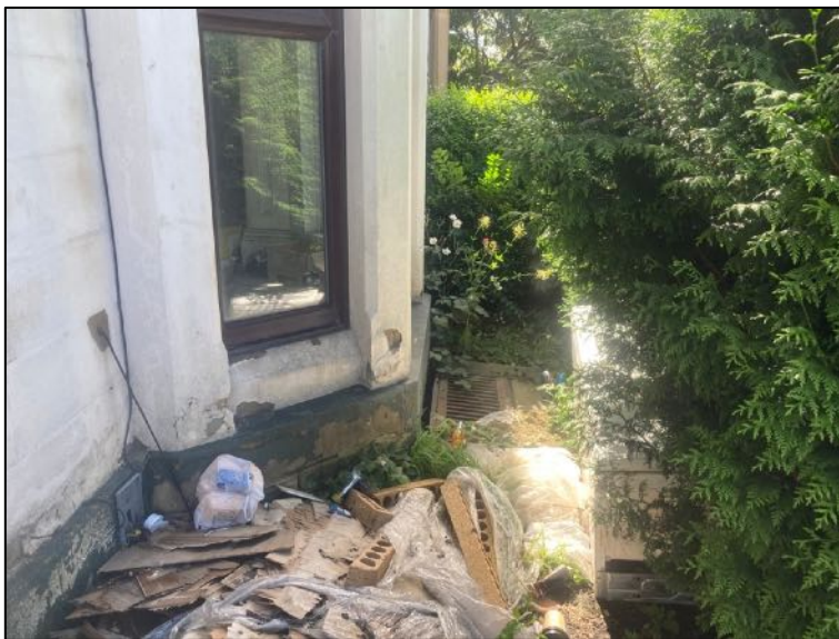
View showing the basement light well with a cast iron grill cover
