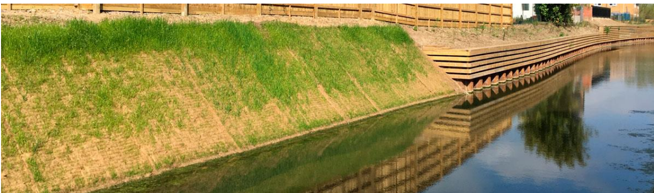
Example of grass growing through coir matting
