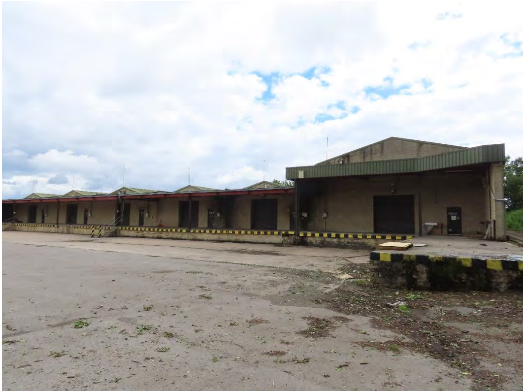
Photograph 8: Large Warehouse building
