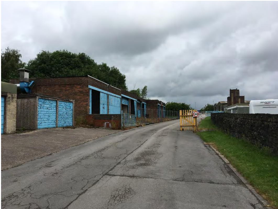
Photograph 3: Tarmac access road and garage buildings
