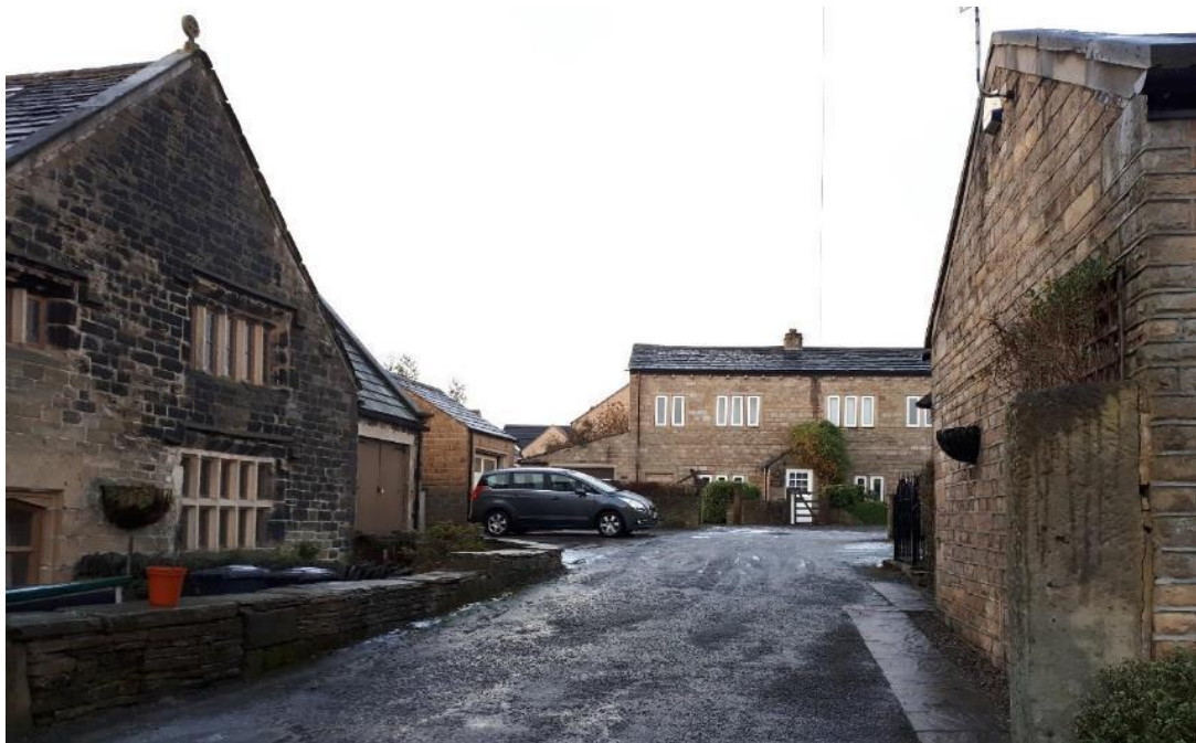
Plate 3: View from Farmhouse Court, looking west toward Crosland Hall Cottage, with the back of Crosland Hall to the left, and the farm buildings to the right of the image
