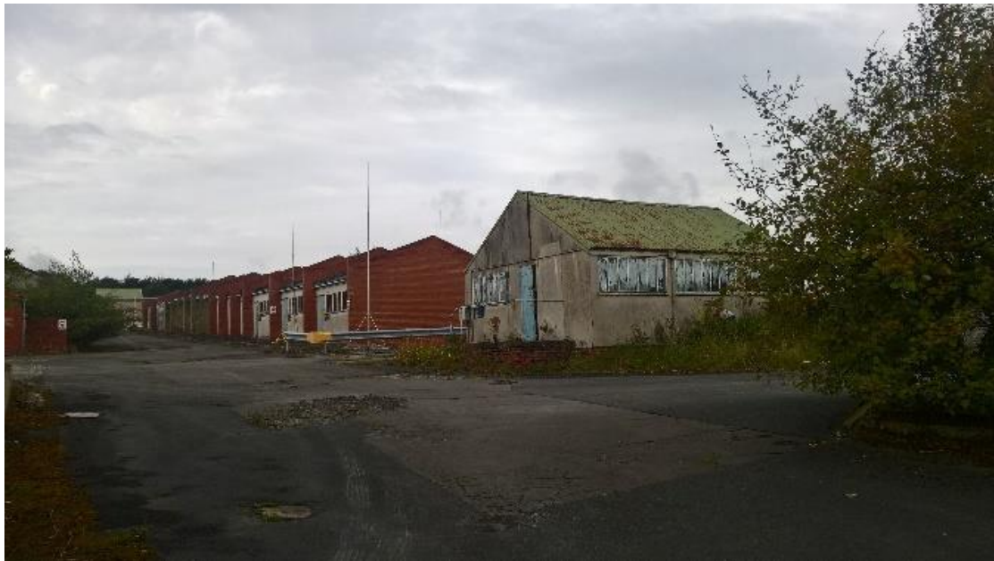
Plate 18: Storage and production units
