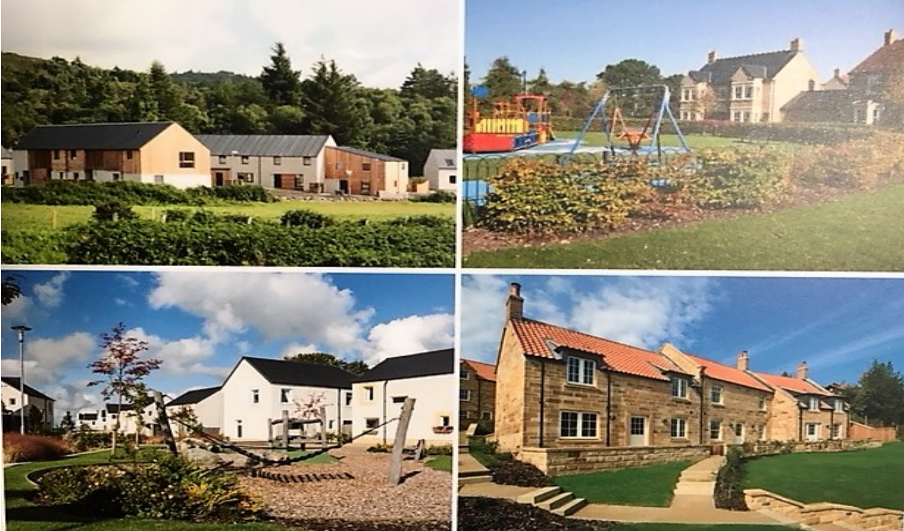
Figure 2.3 Schematic diagrams of proposed buildings and facilities (courtesy of public consultation documents)
