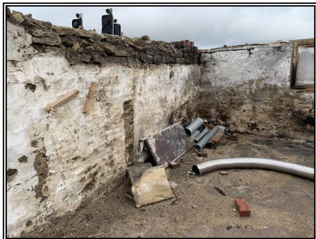
Photo 6: West gable elevation to barn carefully demolished following lightning strike.
