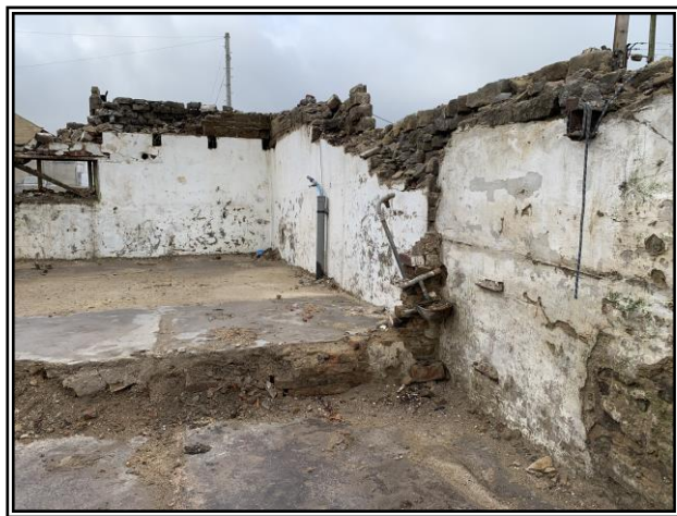
Photo 5: West gable elevation to barn carefully demolished following lightning strike.
