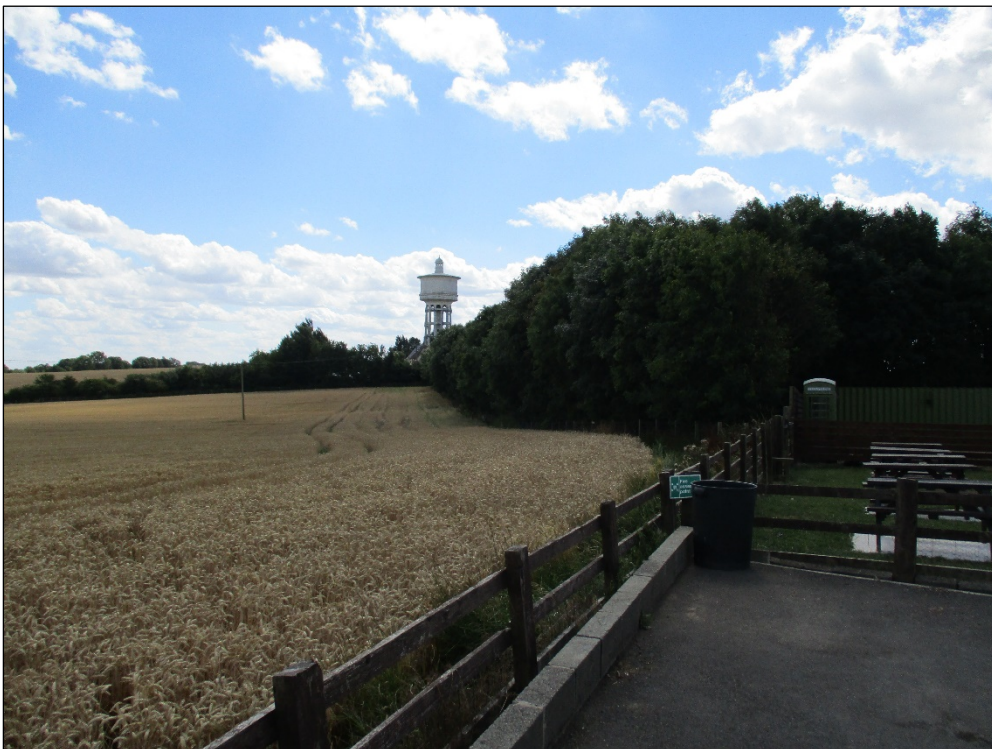
Photo 3: The water tower viewed from the south-western edge of the Site and the beer garden of The Huntsman Public House
