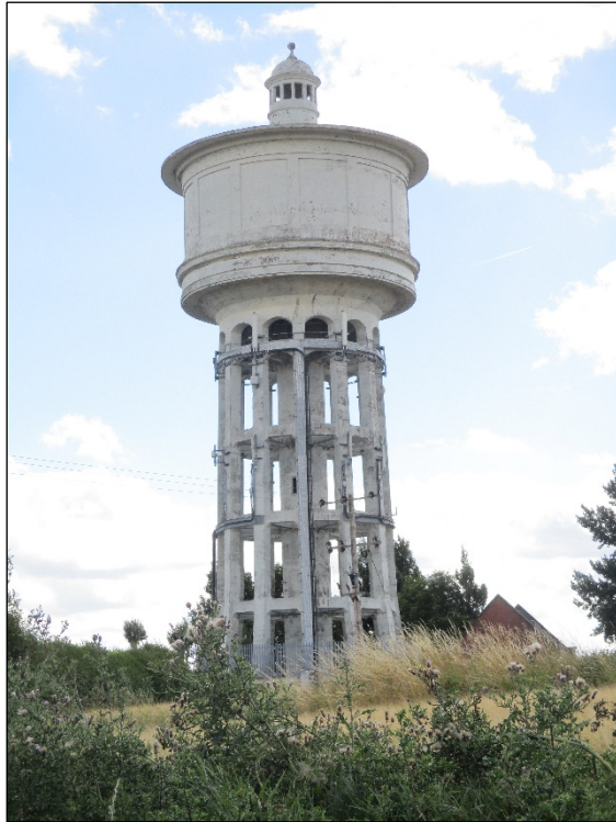
Photo 1: The Grade II Listed Gawthorpe Water Tower viewed from the north-east
