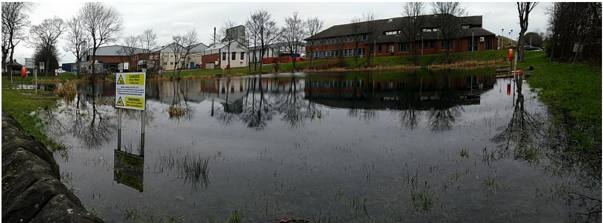
Figure 3 View of pond 5
