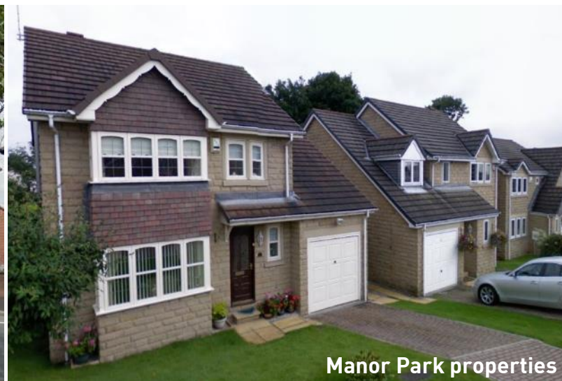
Existing dwellings to Leeds Road
