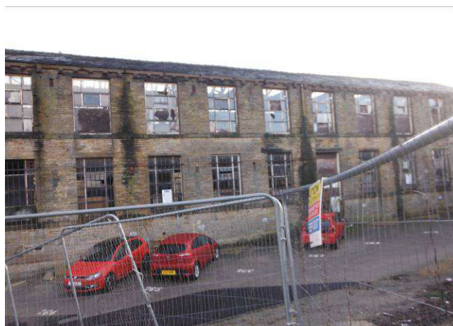
Photo 8: Derelict mills across the road.
