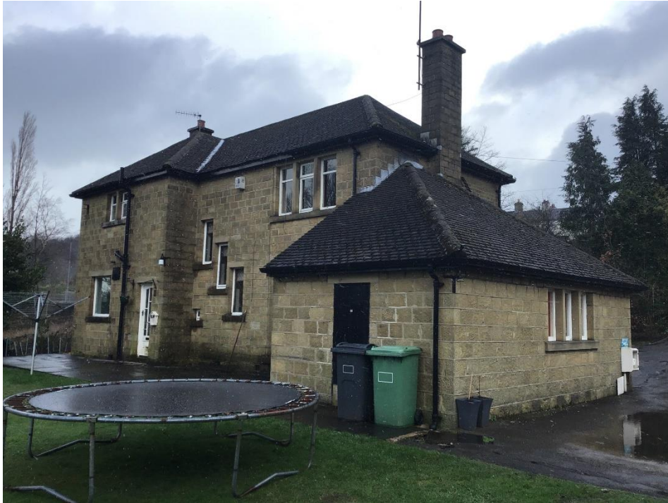
Plate 5. Building 1, viewed from southwest
