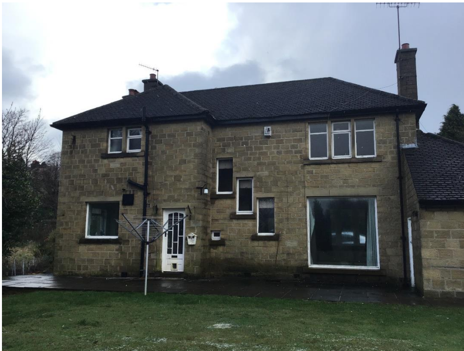
Plate 6: Building 1, viewed from west
