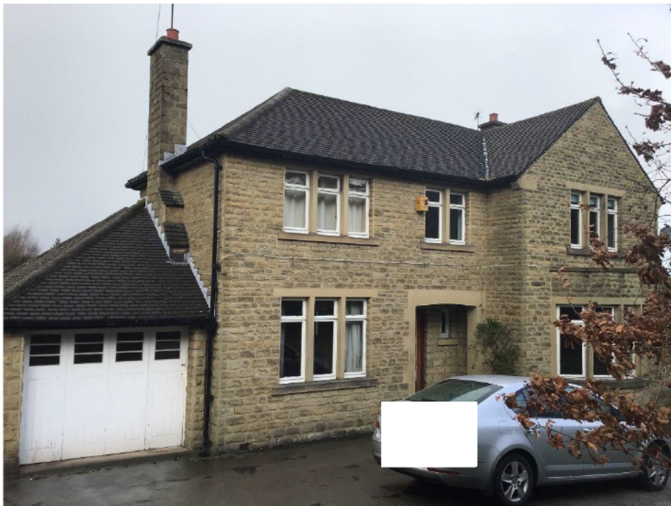
Plate 8: Building 1, viewed from east
