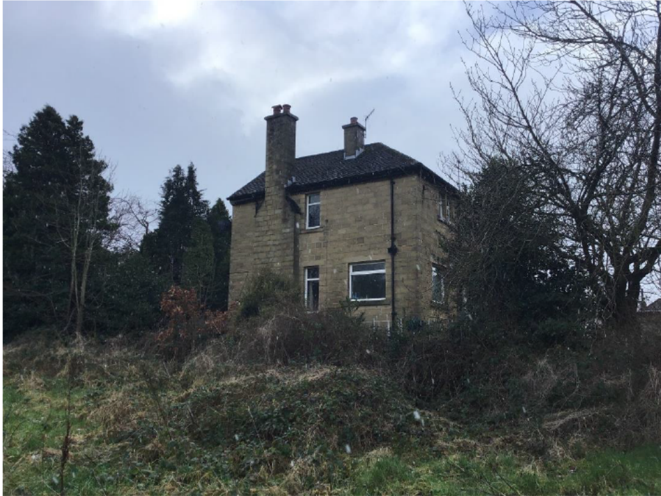
Plate 7: Building 1, viewed from north
