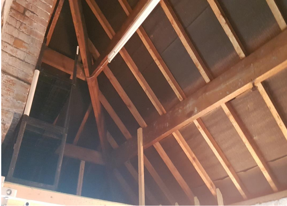
Plate 9: Interior of garage
