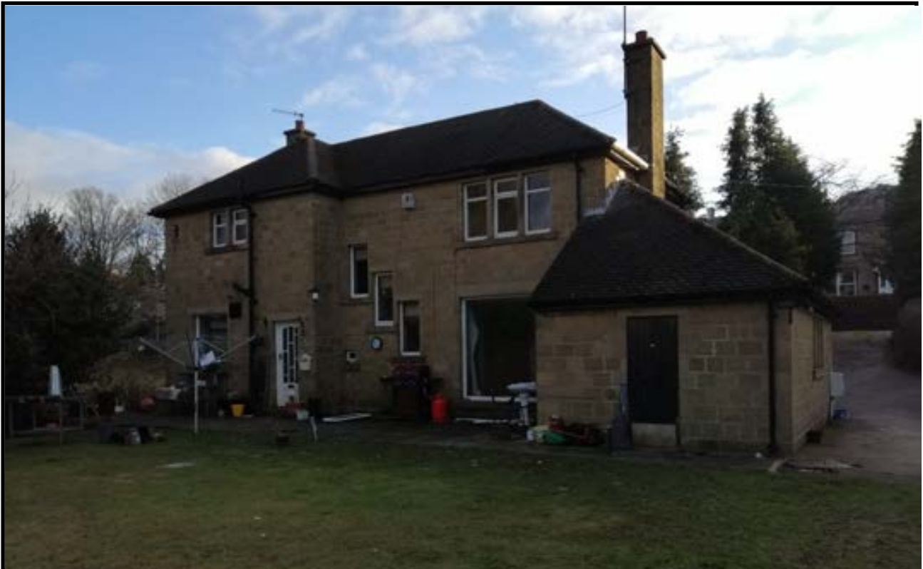
Rear of the property (Facing east)
