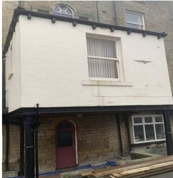
Photo of Rear Toilet Block
