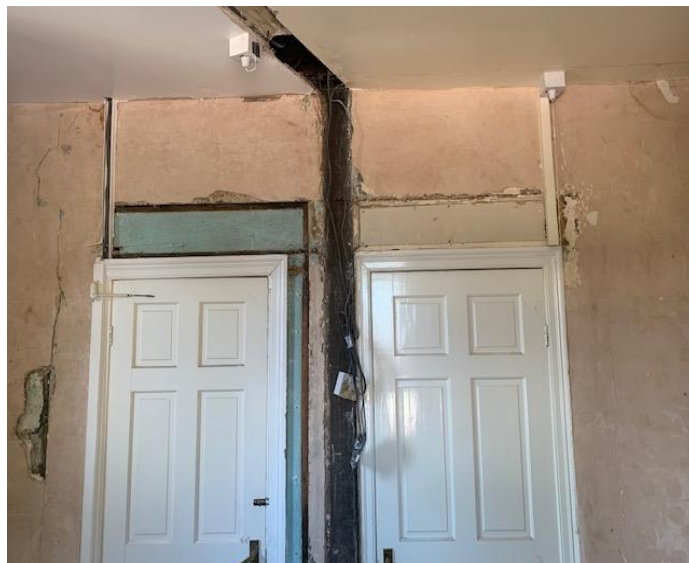
Photo of internal Doors Openings within Rear Toilet Block and previous false wall division
