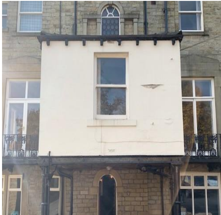
Photo showing Rear Toilet Block covering first floor feature Arch Window
