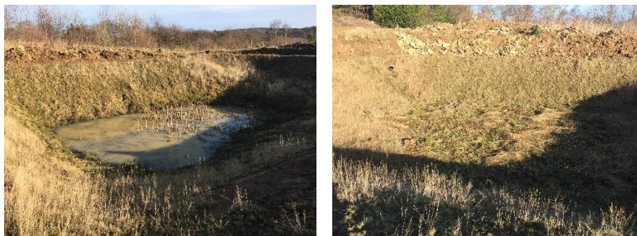
Photograph 9—Pond 1 (left) and Pond 2
