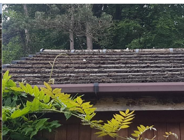
Bungalow, roof tiles
