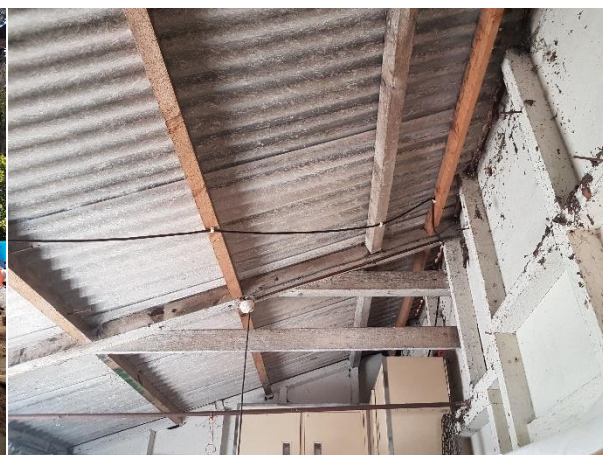
Garage internal roof
