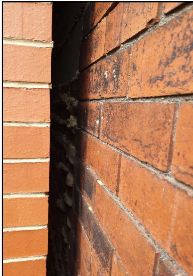
Photograph 5. Rear elevations of 260 - 262 Wakefield Road and 258 Wakefield Road
