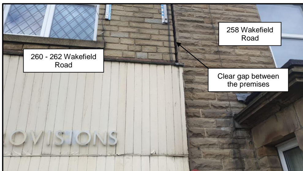
Photograph 4. Front elevations of 260 - 262 Wakefield Road and 258 Wakefield Road
