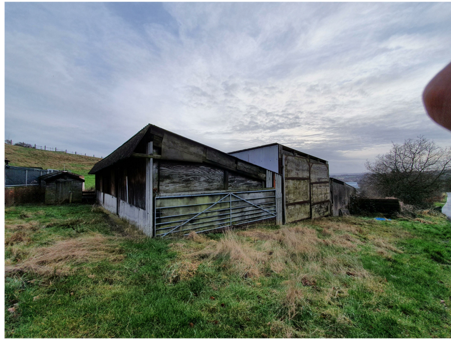
Image - Existing Barn
