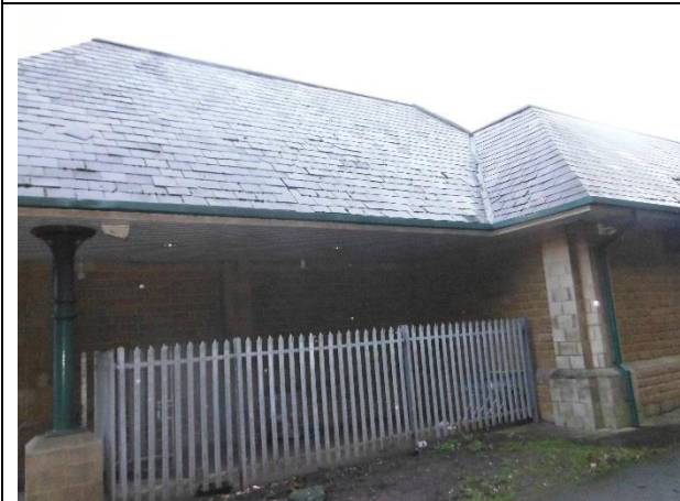
Photo 9: Area to east to be made into indoor floor space.
