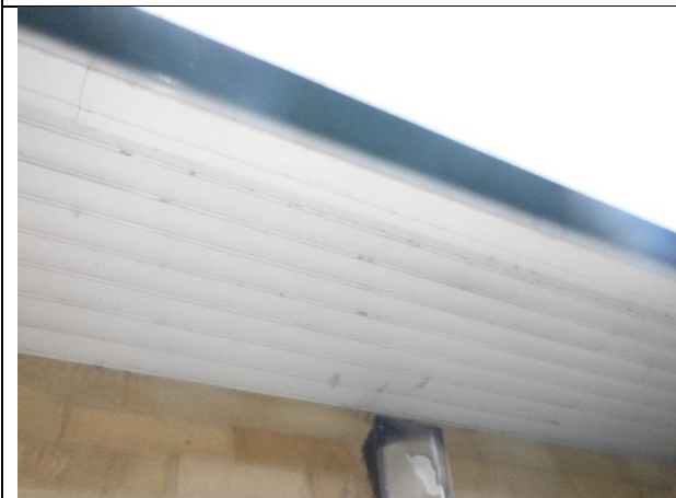
Photo 11: Metal panelling underneath overhangs on the store roof.
