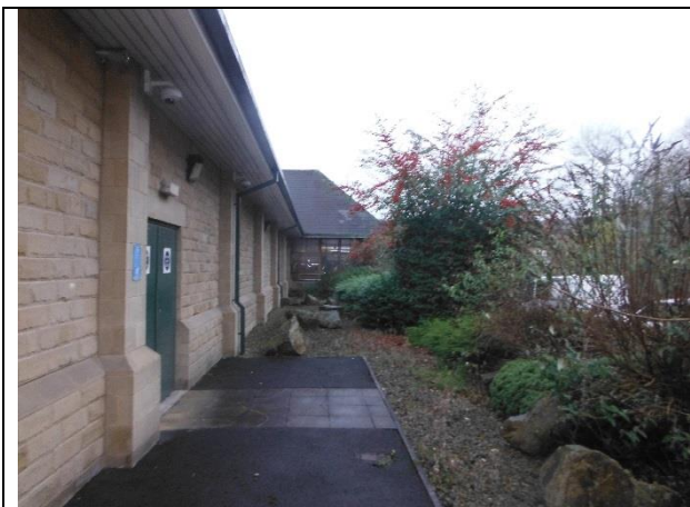
Photo 1: View from the east looking west to side of store to be developed.
