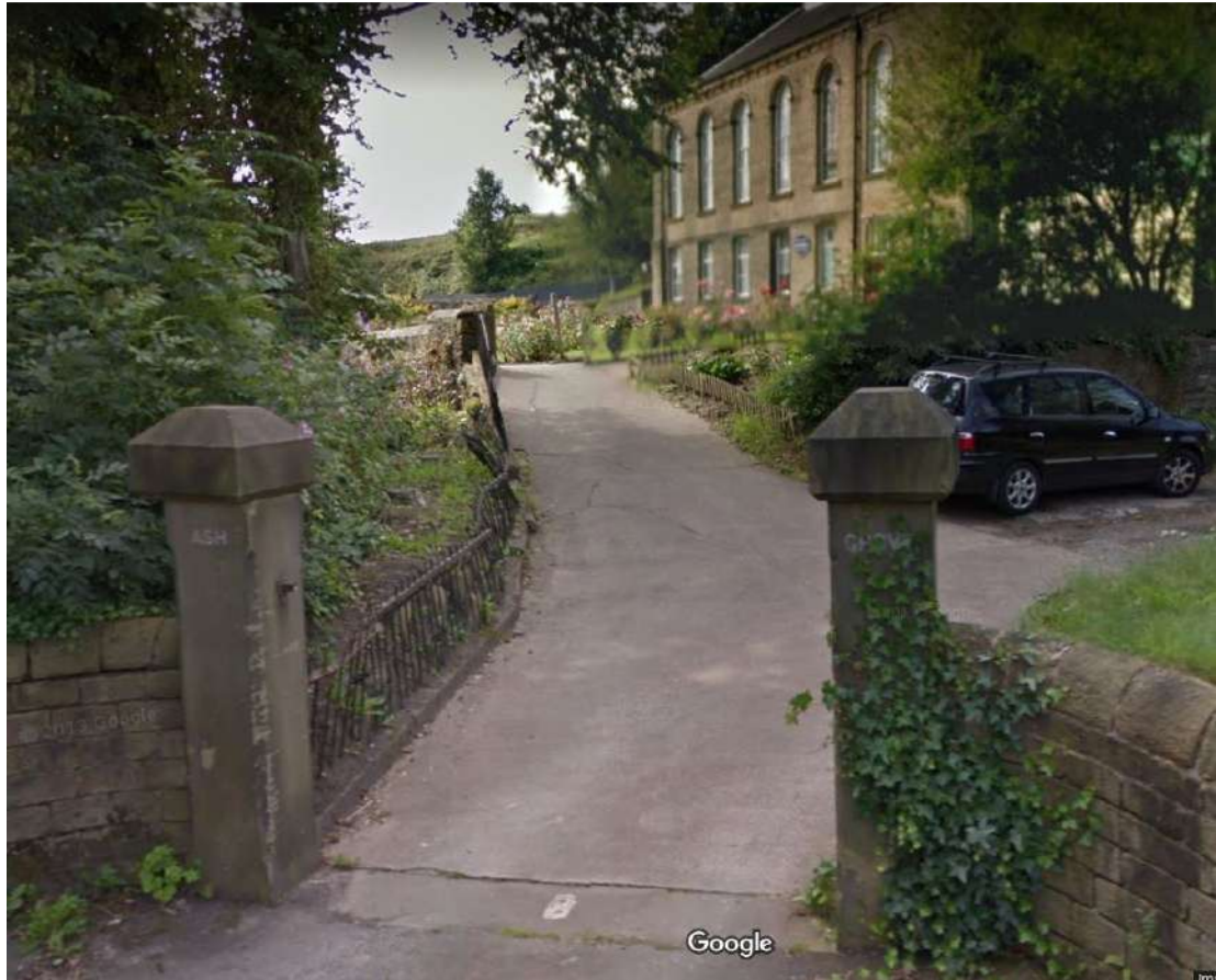
Existing Ash Grove Gate Posts
