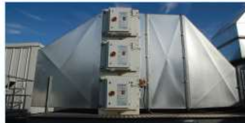
3 ESP Units Stacked in modular formation
