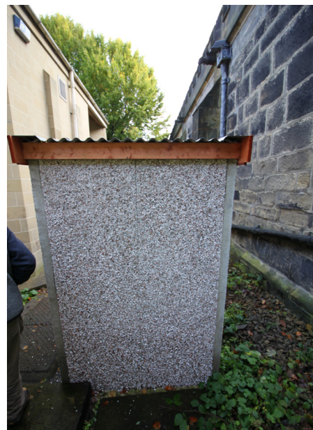
West elevation photo
