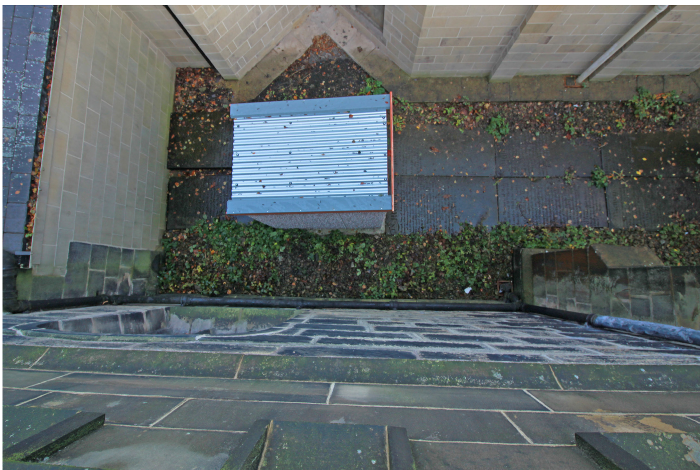
Roof Photo (from the aisle parapet)
