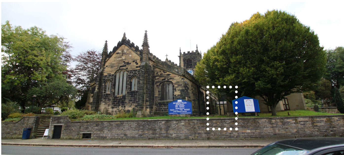
Shed as seen from Northgate, behind the fence
