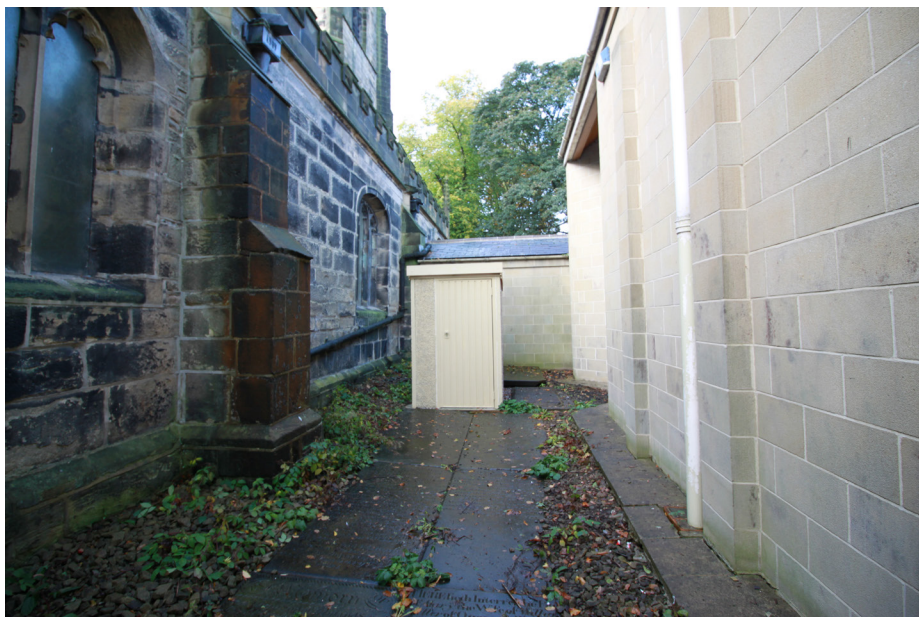
East elevation photo
