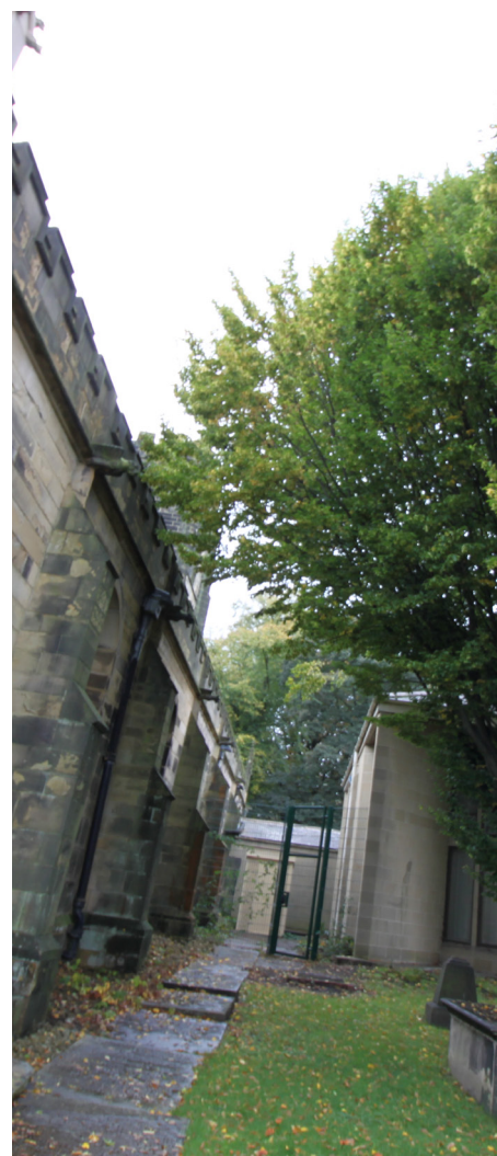
Shed in context, from the Church yard.
