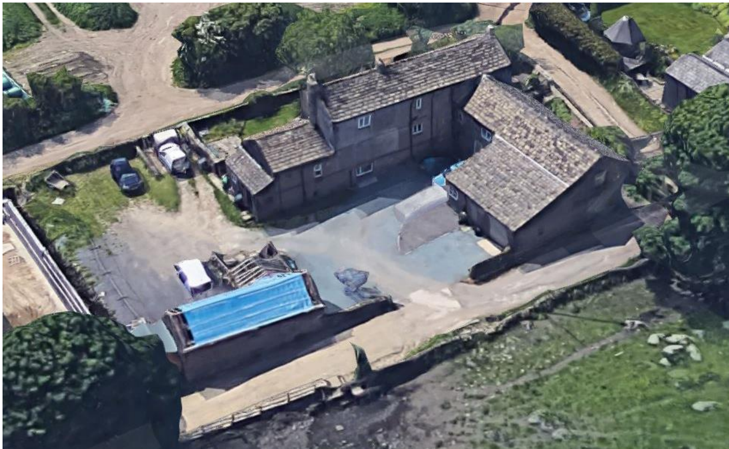
Existing aerial of the Mistal within its setting.
