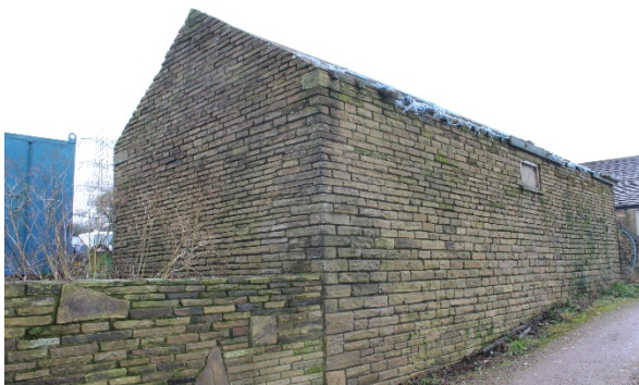
Plate 8 – View of east and north elevation of The Mistal.
