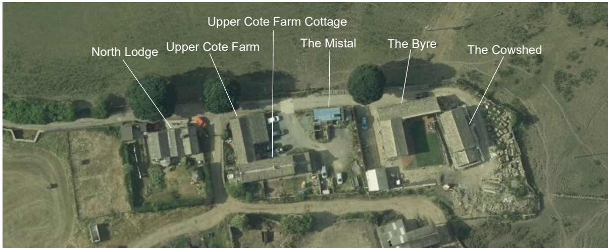
Plate 2 – Aerial view of the buildings at Upper Cote.
