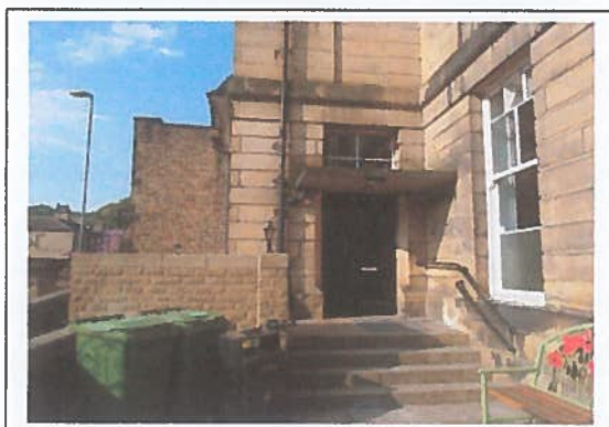
View of the main entrance
