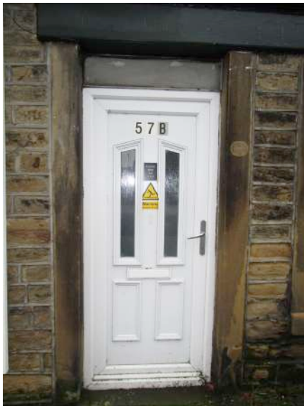
Existing uPVC door.
