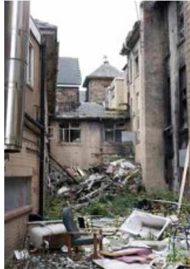
PLATE 8: Batley & District Cottage Hospital Rear elevation showing later infill extensions.
