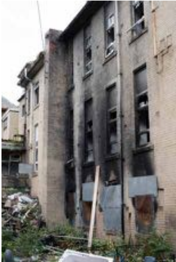
PLATE 7: Batley & District Cottage Hospital Rear elevation of 1920s ward block showing use of brick facing.
