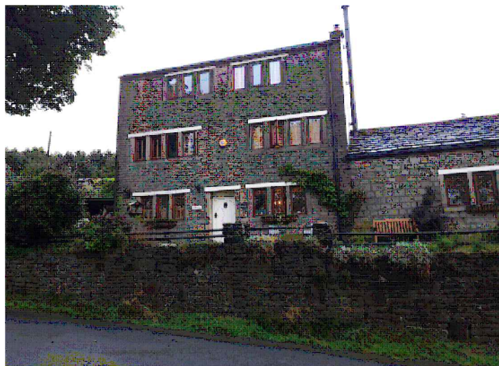
Photo 1 - Front of house
