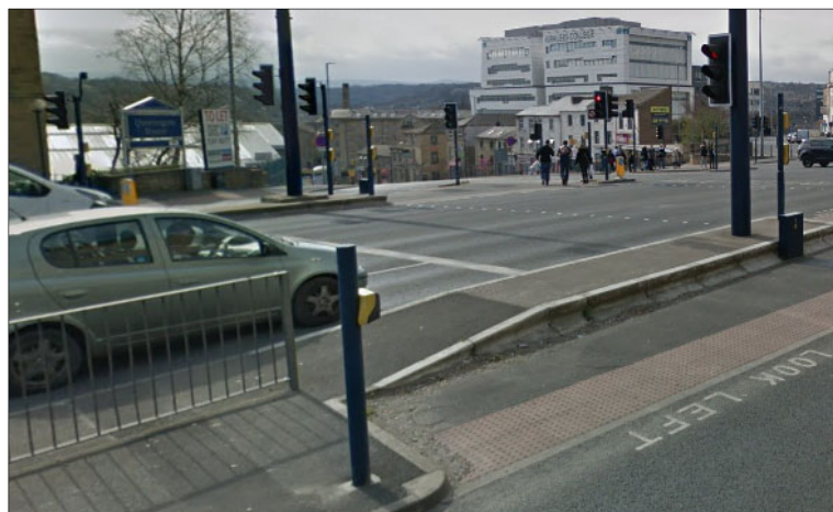
Figure 3.1: Pedestrian Facilities at the A62/A616 Signalised Junction
