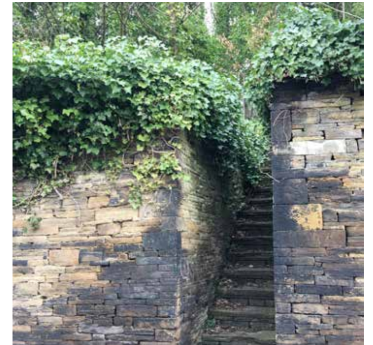
Step access to overcome retaining wall from Ashbrow
