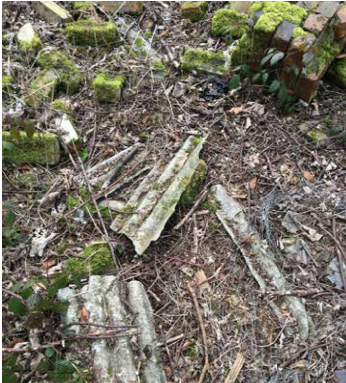
Asbestos roofing tile
