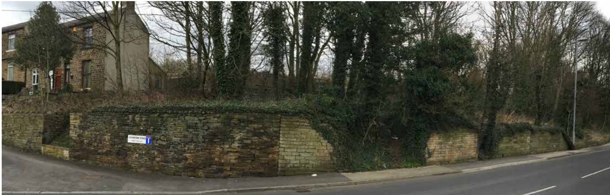
Looking north east up Ashbrow Road – southern site corner foreground
