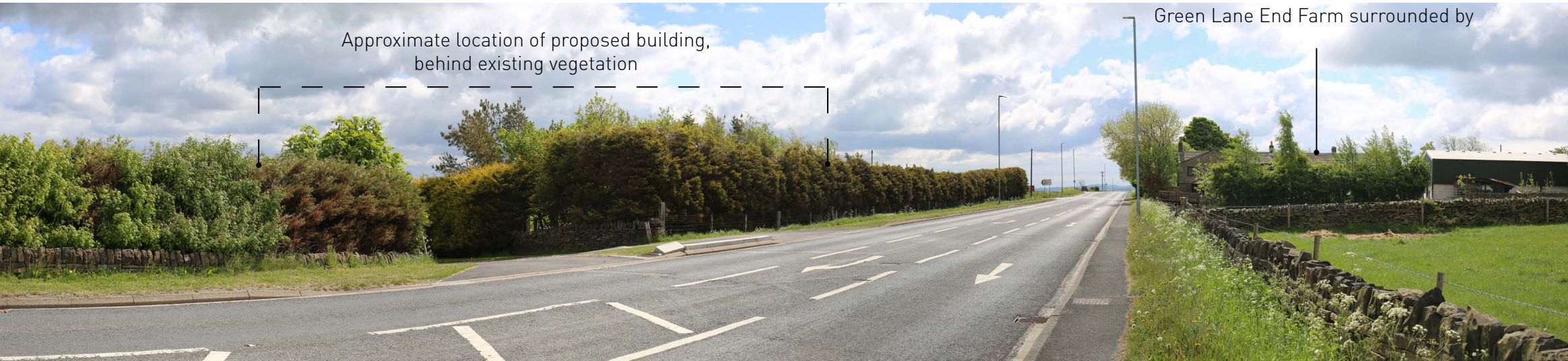
VIEWPOINT 2: FROM PENISTONE ROAD (A629), LOOKING SOUTH-EAST TOWARDS THE SITE
