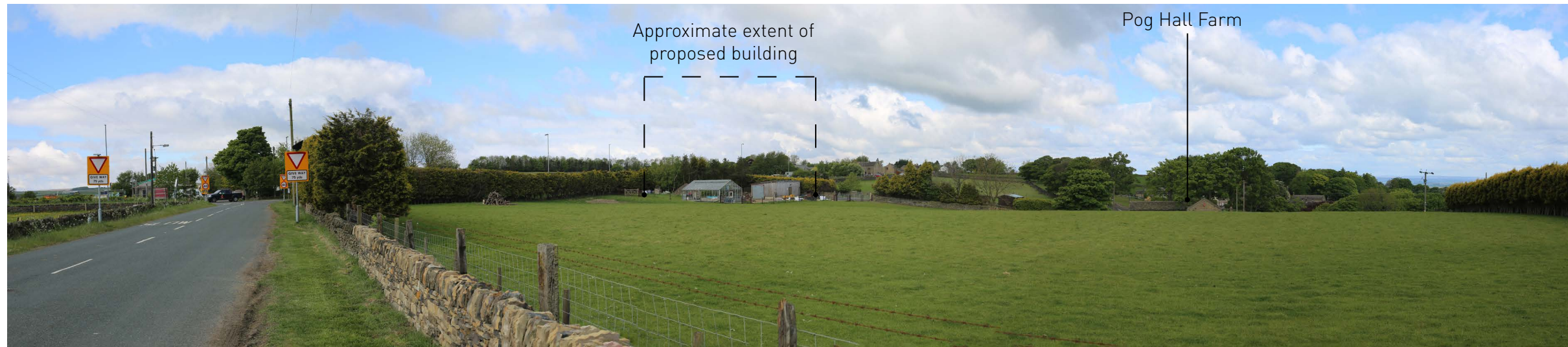
VIEWPOINT 4: FROM DENBY LANE, LOOKING NORTH-WEST TOWARDS THE SITE
