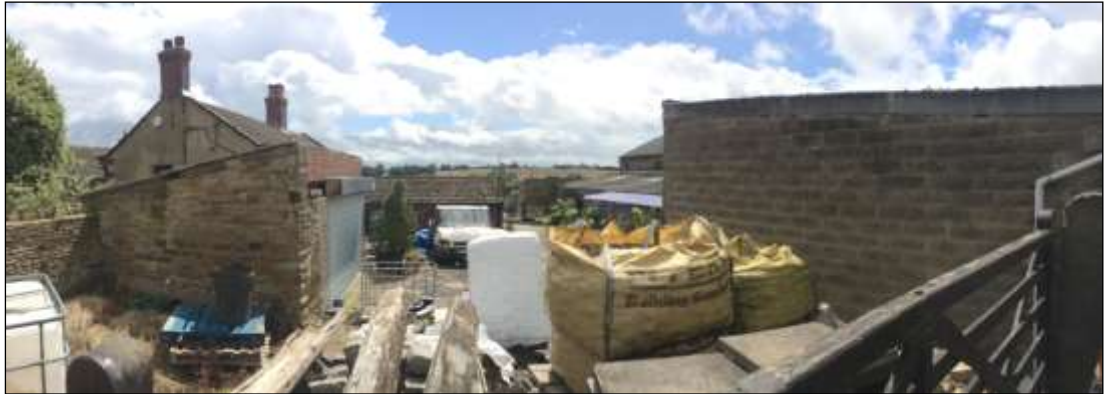
Plate 3. Looking south with Building Section 4 on the right of the image and Building Section 2 on the left
