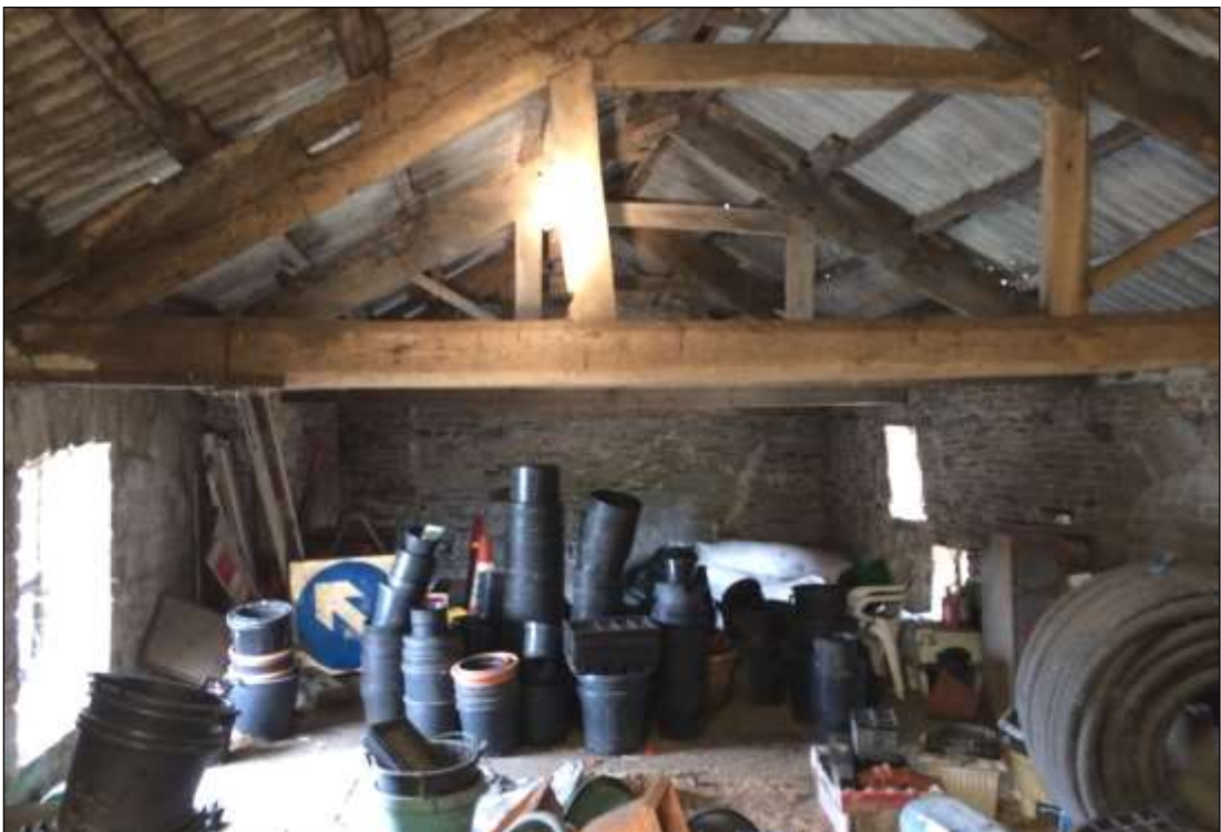
Plate 7. Looking south within the first floor of Building Section 7
