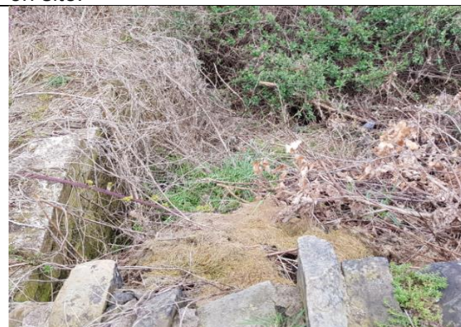
Photo 18: Building foundations on site.
