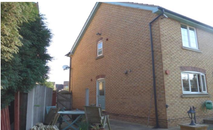
3 East side elevation looking South
