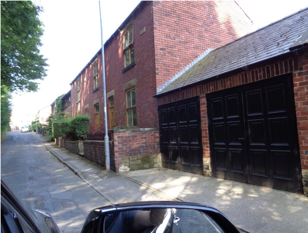
Figure 7: Brick Houses with short building setback
