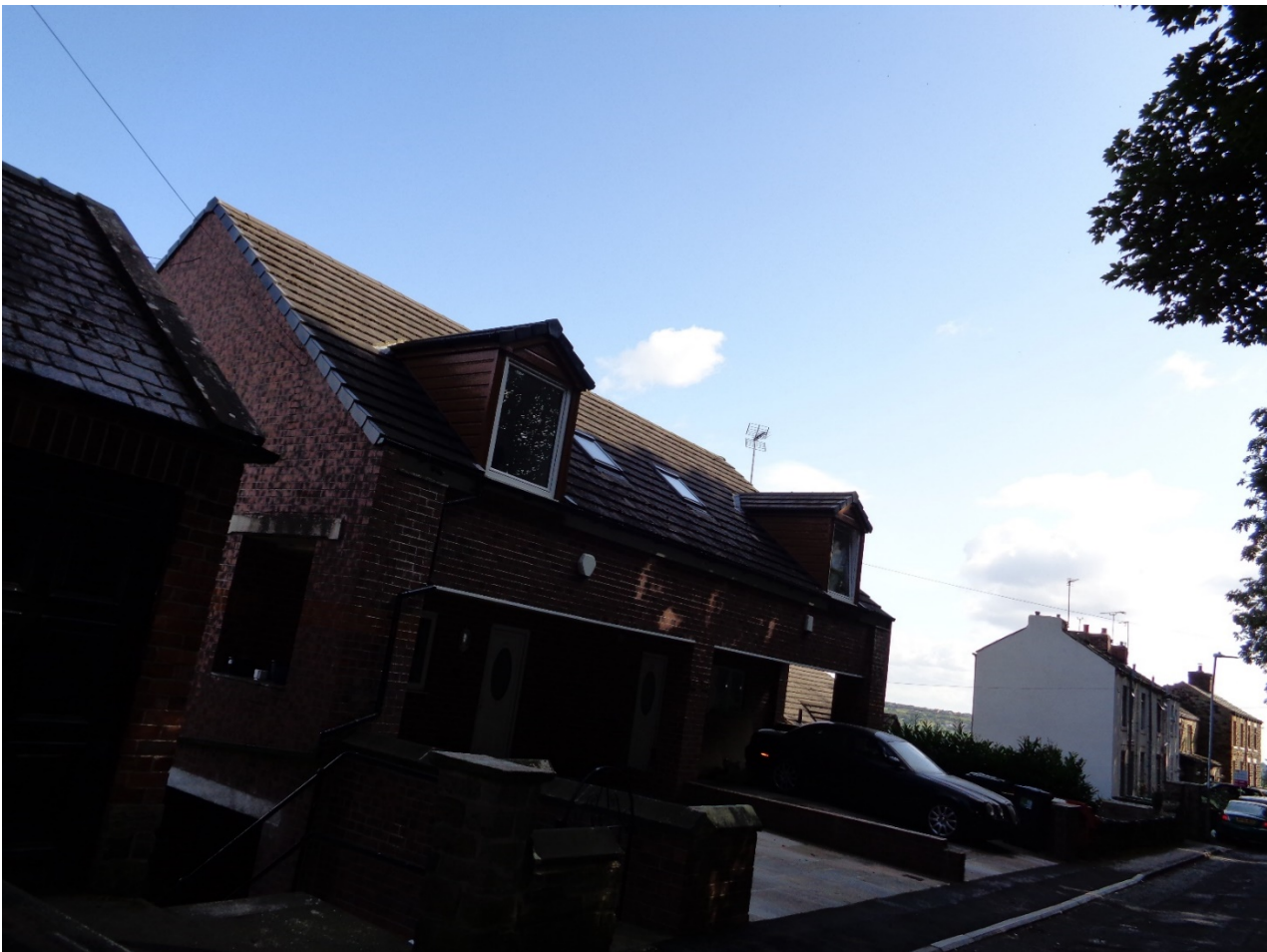
Figure 6: Brick Houses on Wells Road with completely different design than the rest
