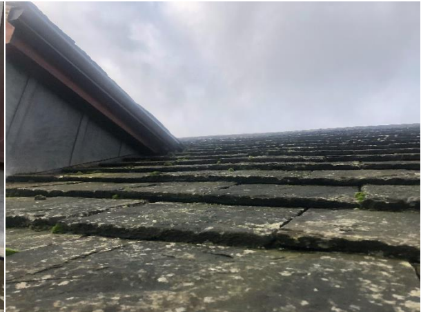
Plate 8. Detail of roof tiles on west aspect
