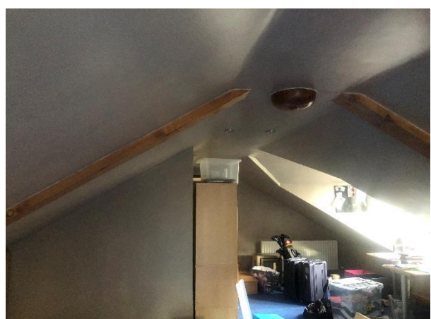
Plate 12. Interior of the upper floor
