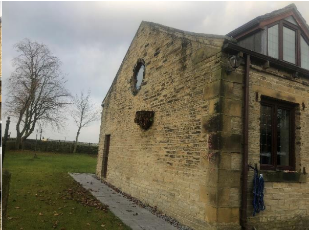
Plate 4. South aspect of the building
