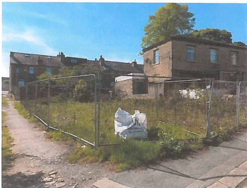
Site as currently seen following demolition of workshop
