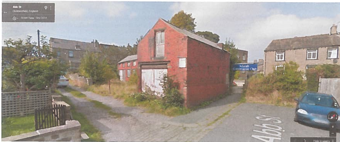
Site as seen prior to demolition of workshop
