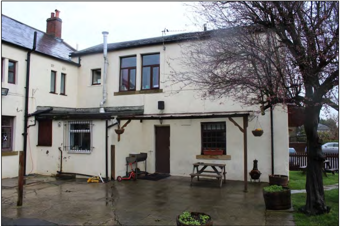
Photo 2: Overview of southern range, looking east
