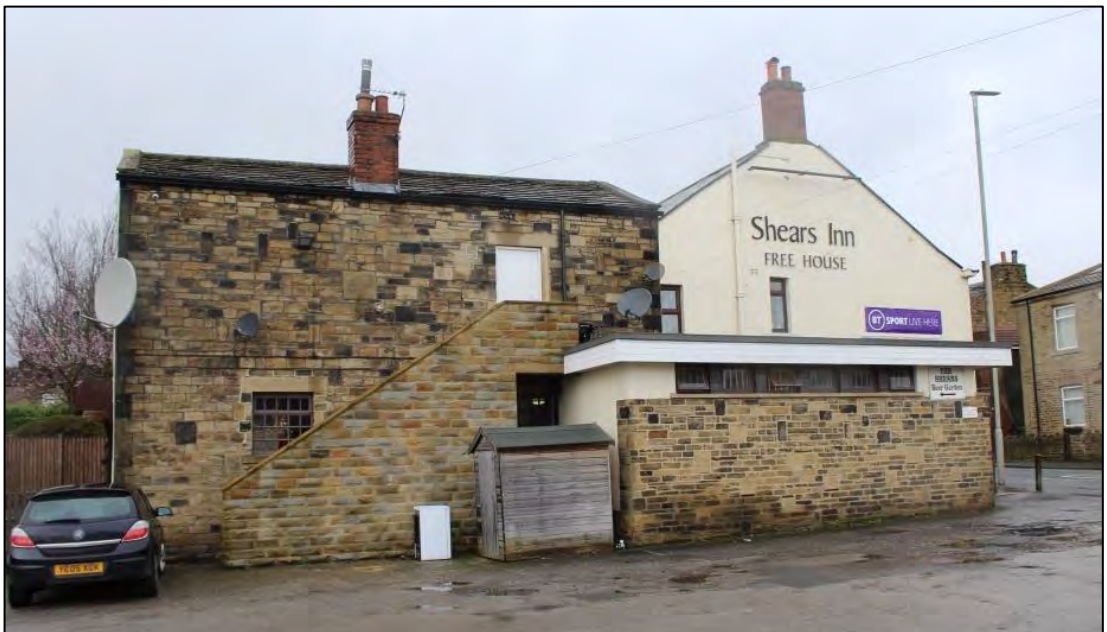
Photo 3: Overview of southern range, looking west
