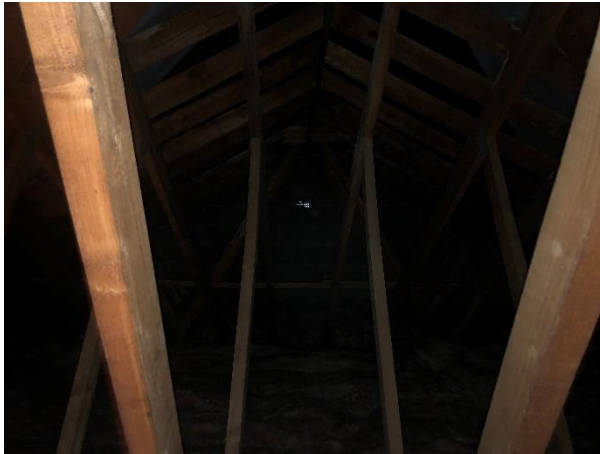
Plate 7 Interior roof void of the building
