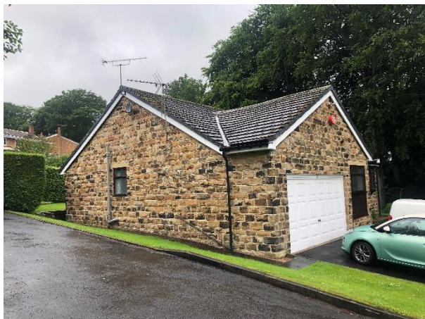
Plate 1 Southeast aspect of the building
