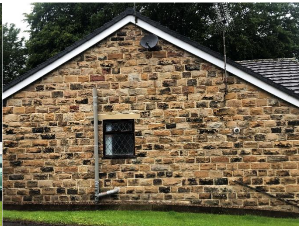
Plate 2 Southeast gable and bat emergence point
