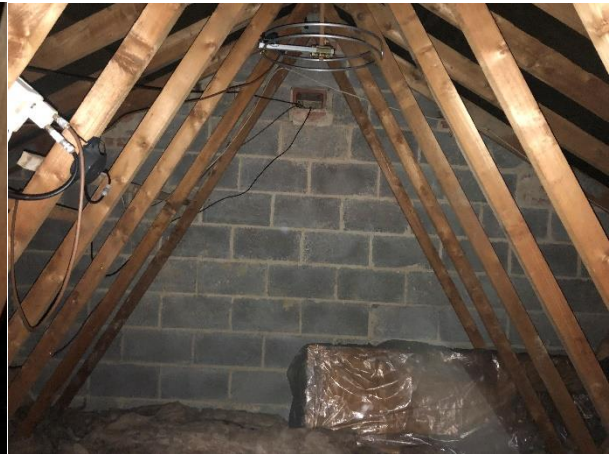
Plate 8 Interior roof void of the building
