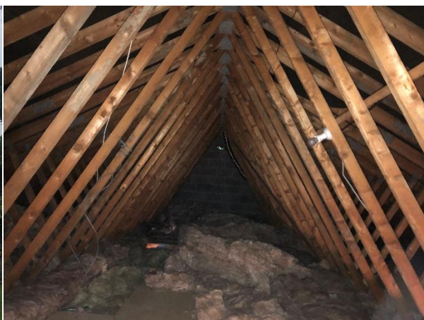
Plate 6 Interior roof void
