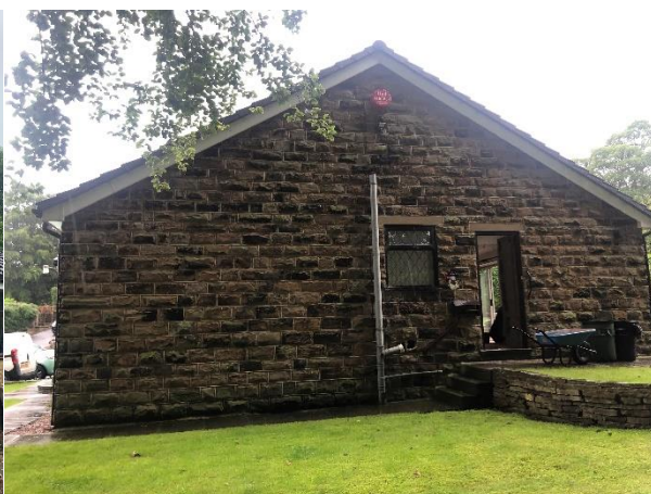
Plate 4 Northwest gable of the building
